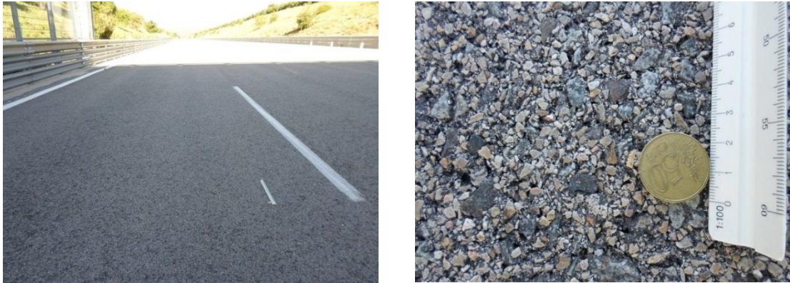
Figure 39: The high-speed circuit and associated asphalt structure
