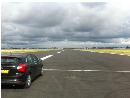
Figure 48: Ambient conditions at the Valkenburg air-strip
