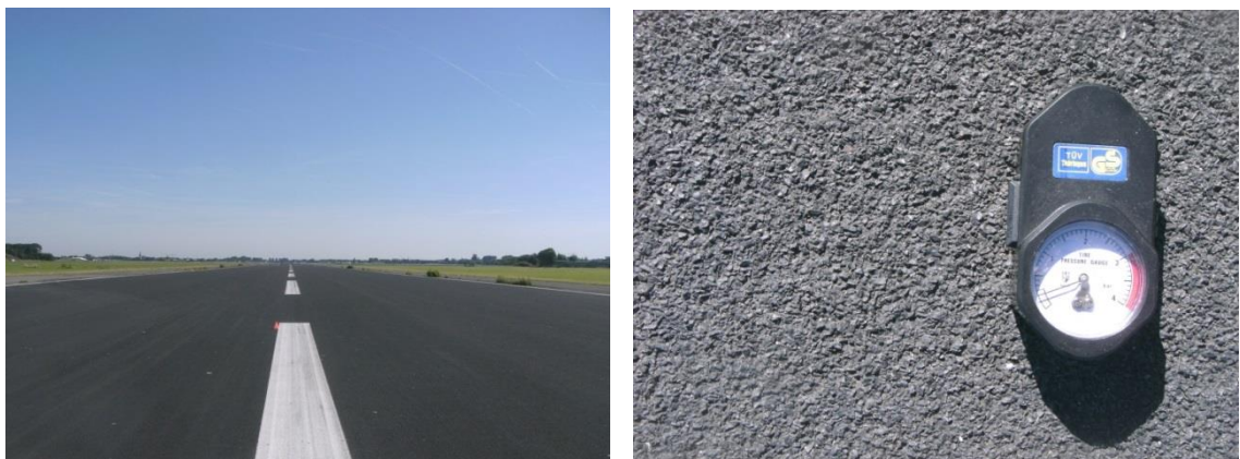
Figure 37: The air-strip and asphalt structure at air base Valkenburg
