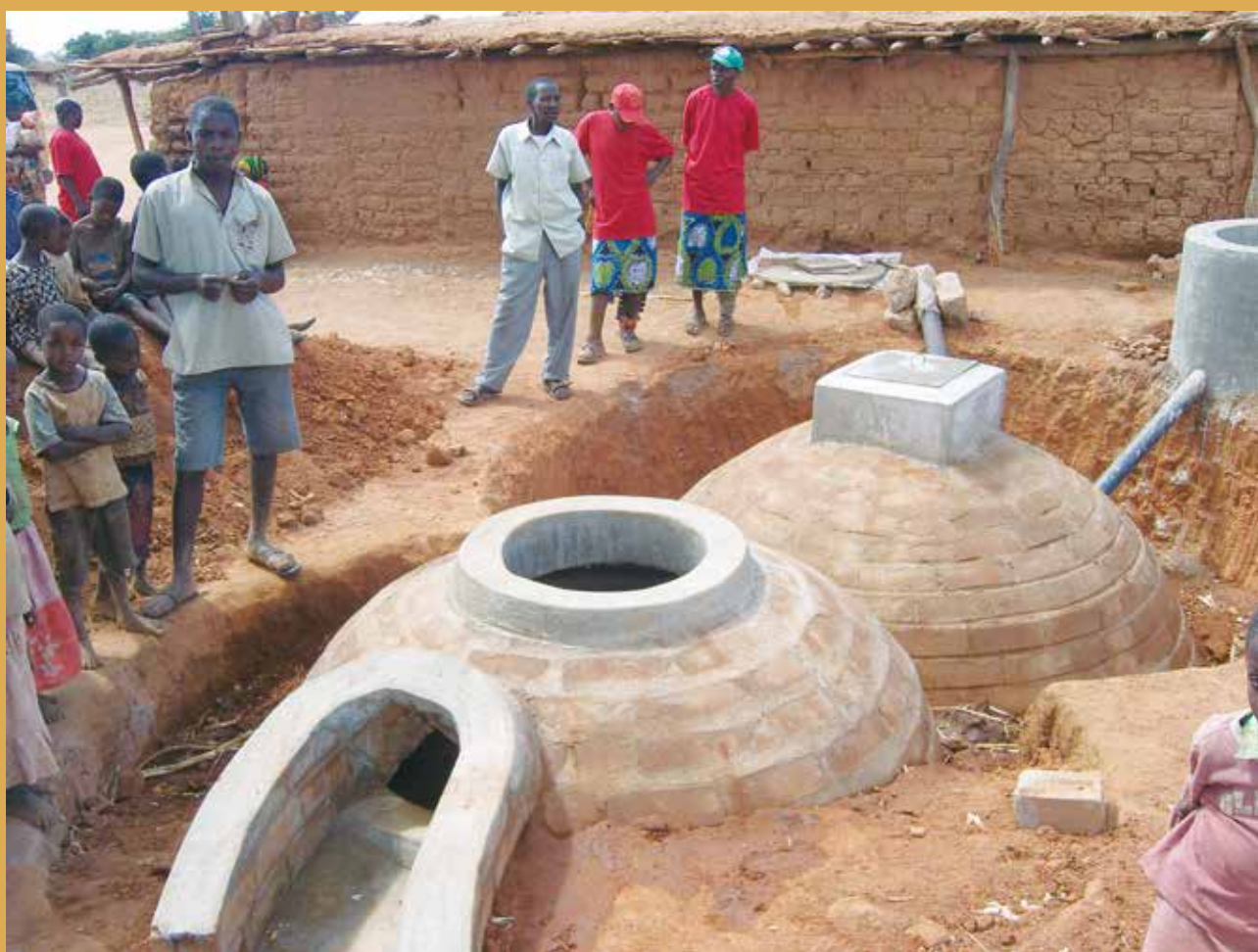
Construction of biogas digester, Chololo eco-village project
