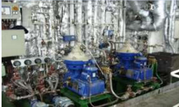
Centrifuges remove water and sludge from the fuel
