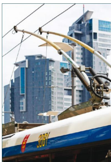
Figure 86: Trolleybus poles (photo by TROLLEY project)
