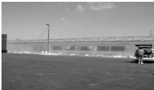
Figure 3: General view of the drier consisting of a green house.
