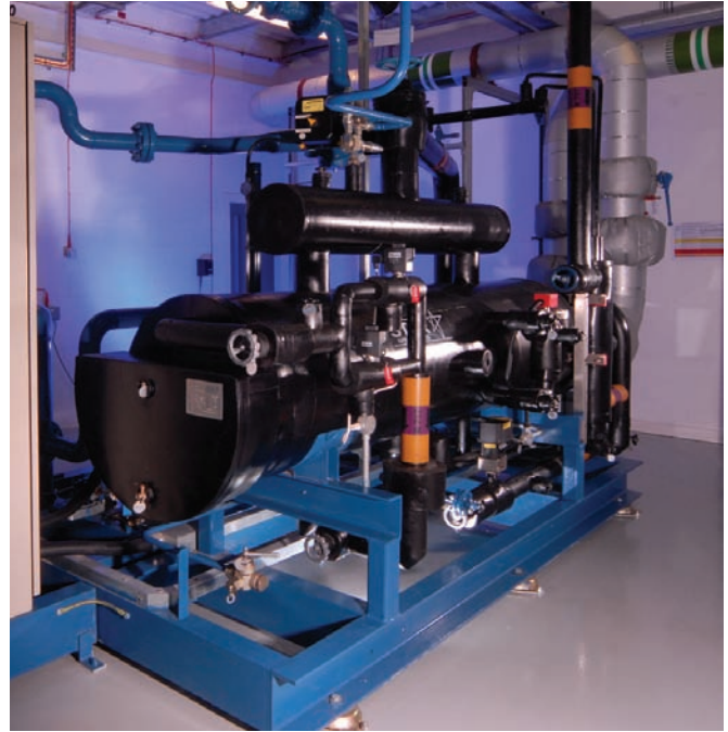
Photo 1 (left): A 2500 kW chiller being installed. Photo 2 (right): Free chillers that use thermosyphon to provide highly efficient cooling.
