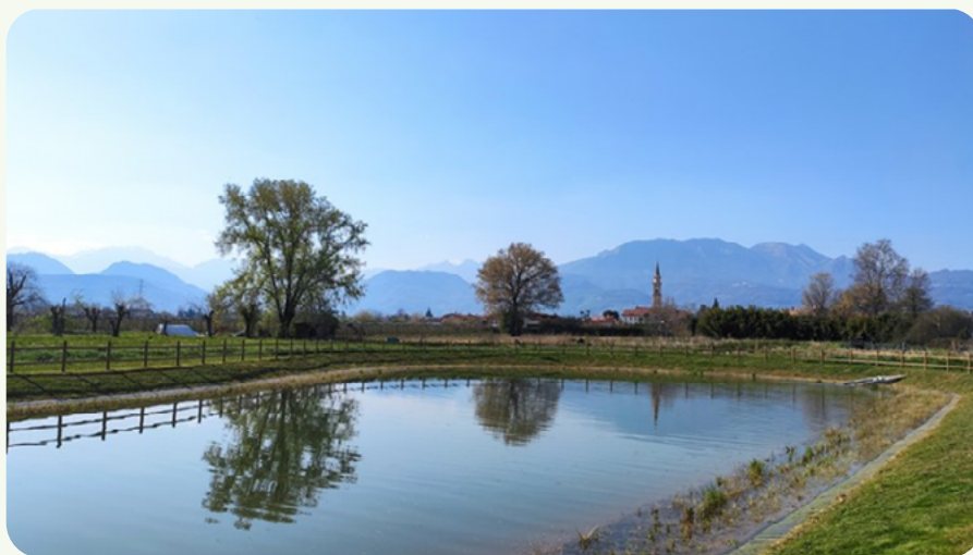
Detention basin after its construction in the agricultural area of Giavenale
