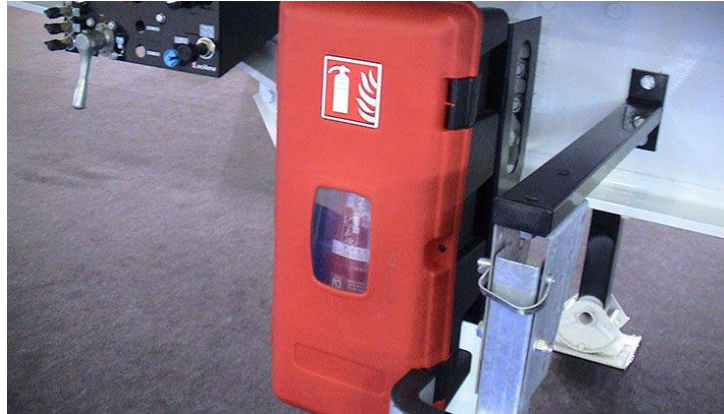
Figure 21: Example of a fire extinguisher mounted inside a box
