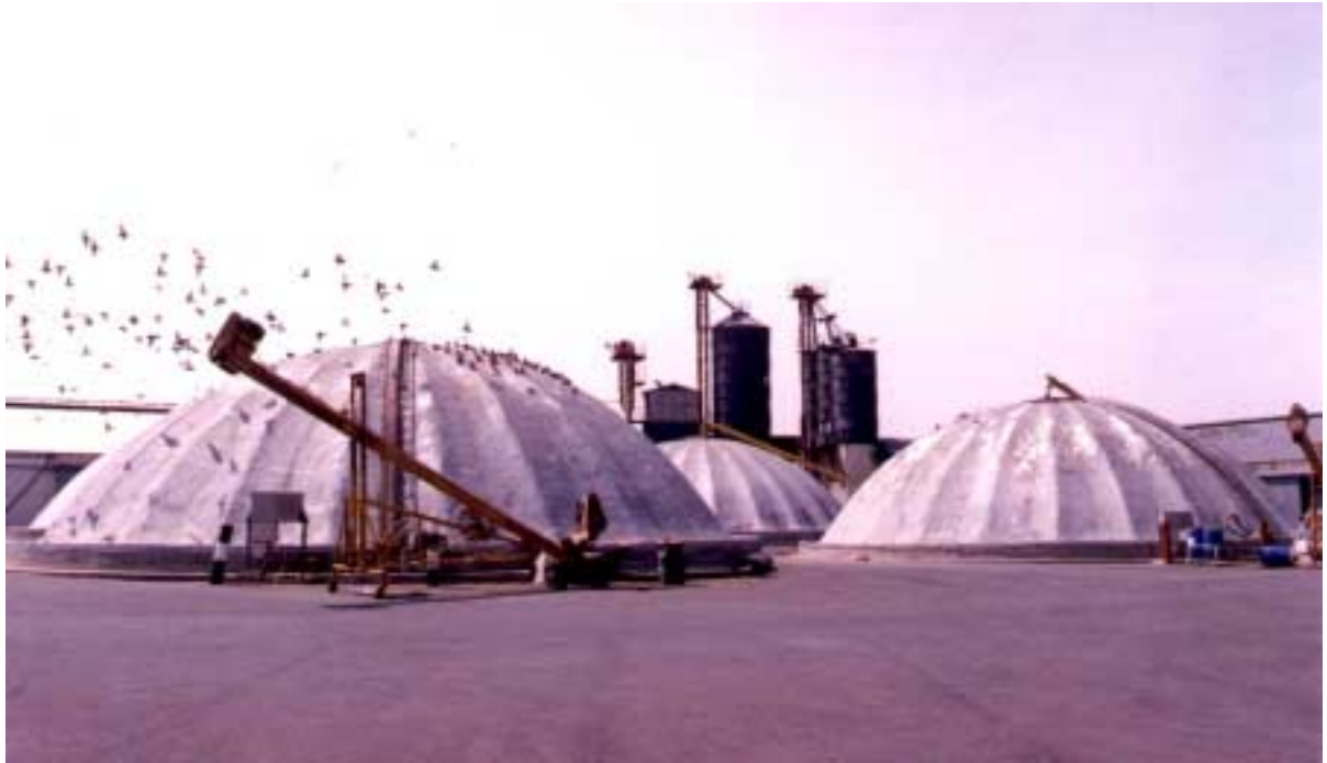
Photo 2: The historic "Cyprus Ctessifon semi-underground pits" built in 1956 and served as an international model for studying the possibility of using hermetic structures for grain storage.
