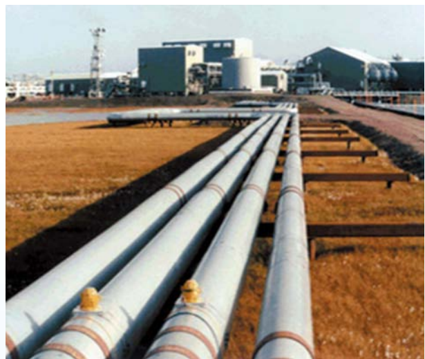
Figure 3.5 More than 2500km of CO 2 pipelines are already in use in the USA for EOR (Courtesy of BP)
