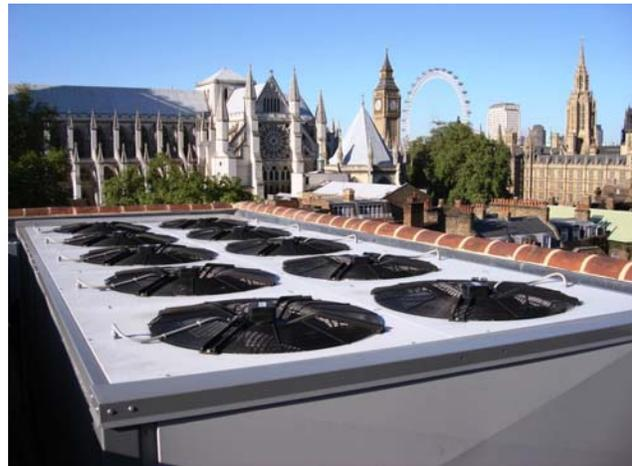
The technical development of the system was straightforward; the most time-consuming element was optimising the selection of compressors, heat exchangers and valves for our more efficient, “non-standard” conditions. The main barriers faced in developing the technology, were initially getting selection data for components using hydrocarbon refrigerants and, more recently, getting components CE marked.<sup>2</sup>
