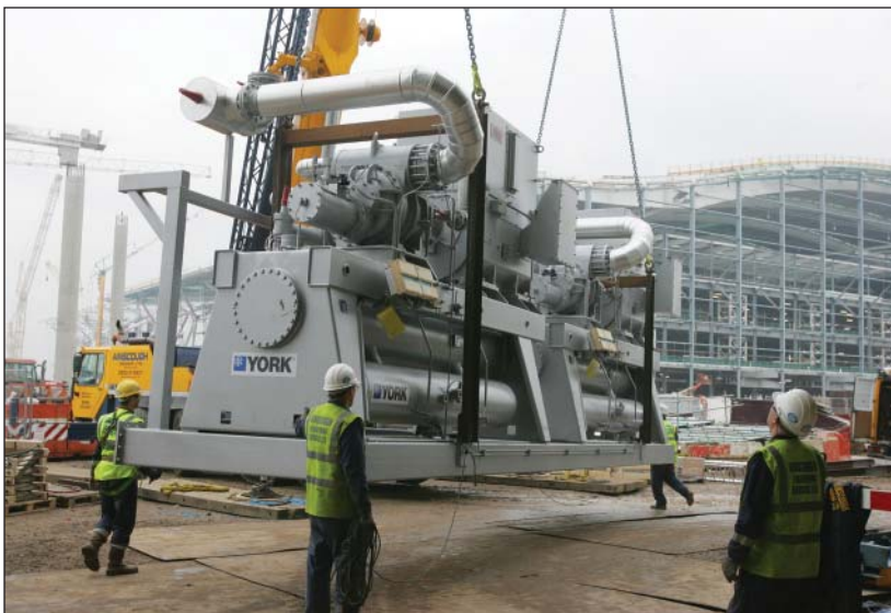
Figure 3: One of four packaged ammonia chillers being installed at Heathrow Airport Terminal 5
