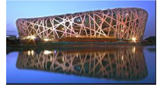
Beijing Olympic Stadium insulated with Huntsman's PU system
