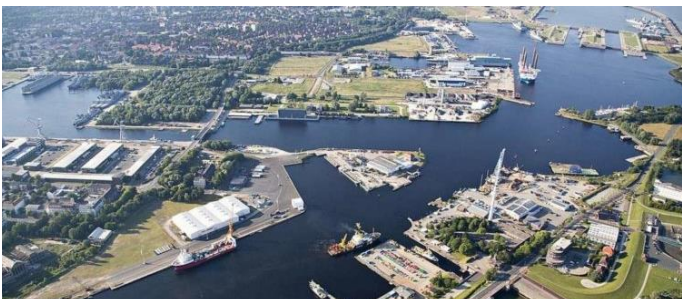
Access to key energy hub Wilhelmshaven, Germany
