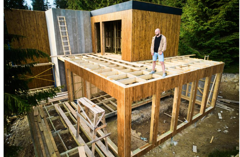
Image: Carpenter constructing wooden frame house. by anatoliy_qlieb , envato elements
