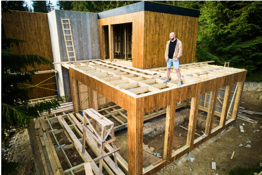
Image: Carpenter constructing wooden frame house. by anatoliy_gleb , envato elements
