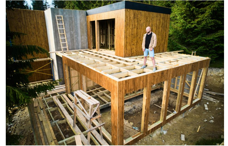
Image: Carpenter constructing wooden frame house. by anatoliy_gleb , envato elements
